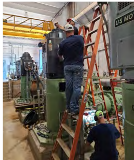
JWC staff re-installing raw water pump
