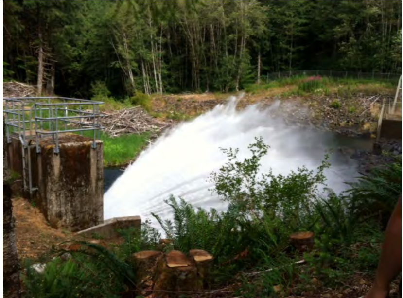
Release from Barney Reservoir to the Trask River through a Howell-Bunger Valve
