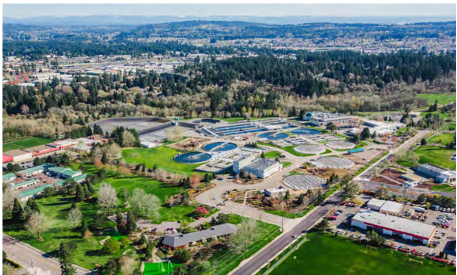
Durham Wastewater Treatment Facility
