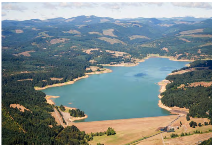
Scoggins Dam and Hagg Lake
