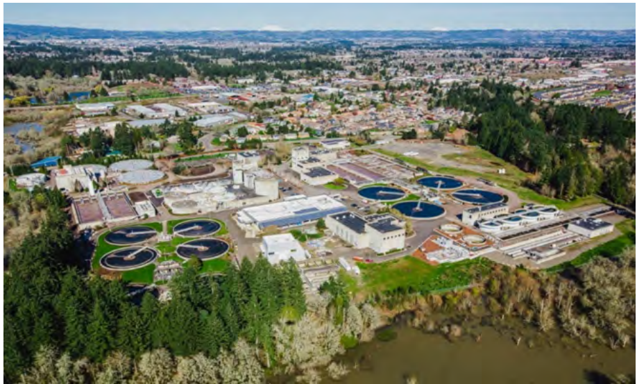
Rock Creek Wastewater Treatment Facility
