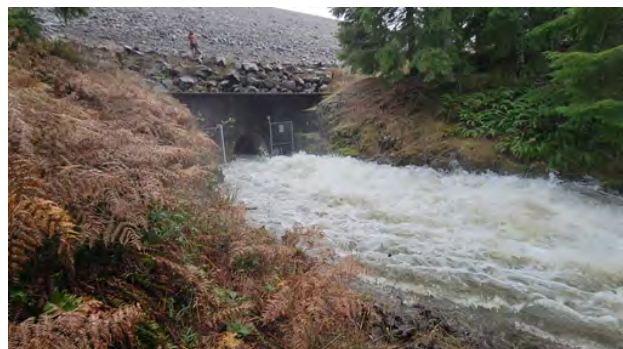
Water from Barney Reservoir via emergency spillway to dissipation area above the Trask R.
