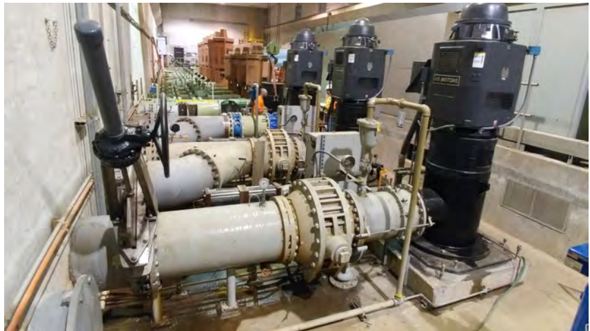
Raw water pumps were replaced
