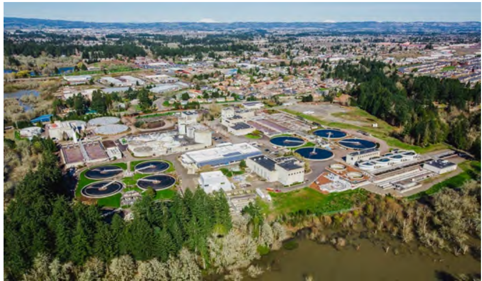
Rock Creek Wastewater Treatment Facility
