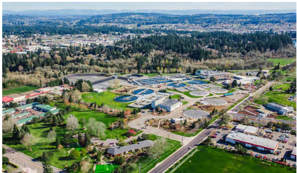
Durham Wastewater Treatment Facility
