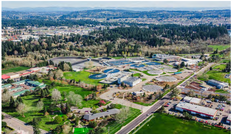
Durham Wastewater Treatment Facility
