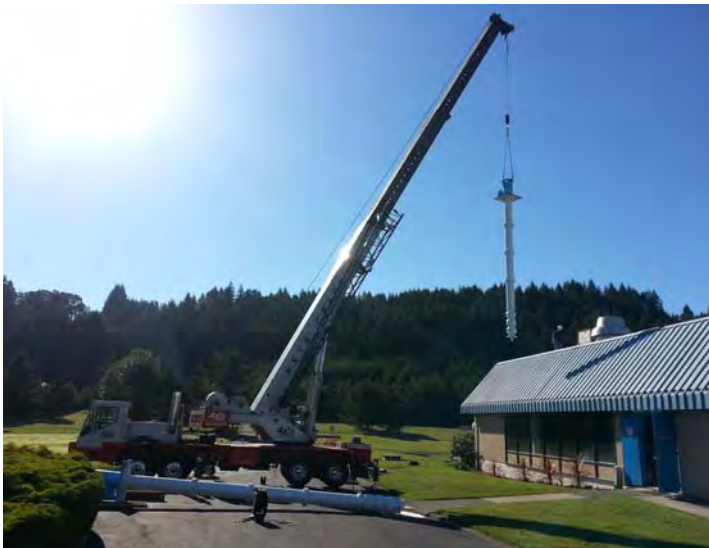
Finished water pump being replaced.
