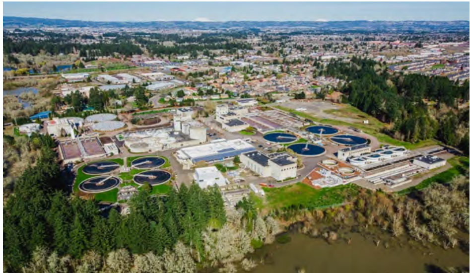
Rock Creek Wastewater Treatment Facility
