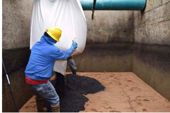
Filter media being replaced.
