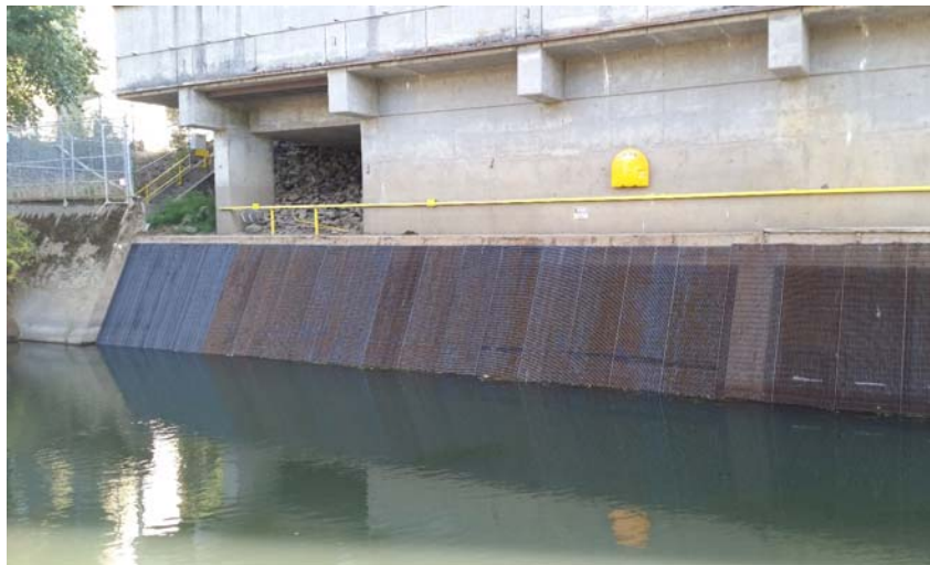
Completed installation of new trash rack bar screens at SHPP
