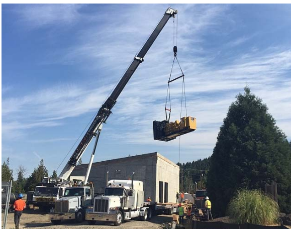
Generator installation at WTP, August 27, 2105
