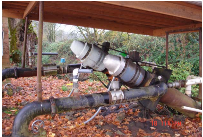
Surface water diversion metering on Gales Creek, a high priority stream for flow restoration.
