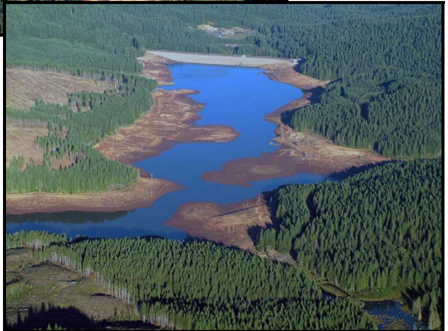
Barney Reservoir, after drawdown, September 2011
