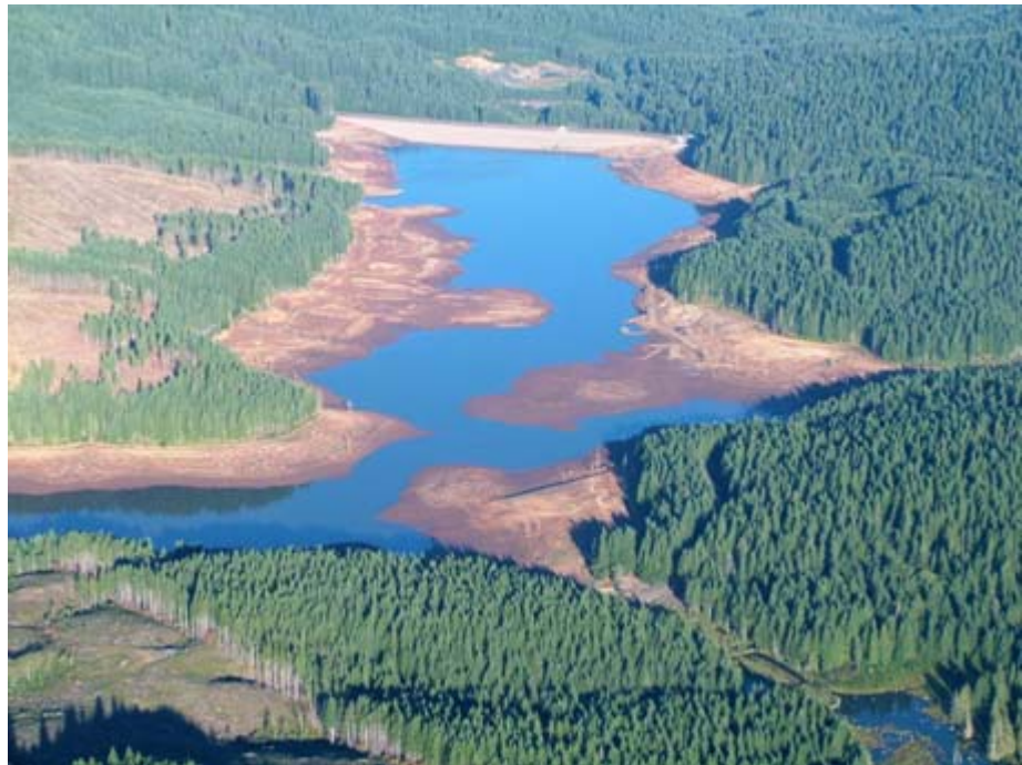
Barney Reservoir drawn down to a surface water elevation of 1,580 ft. At this level, the reservoir contains approximately 2,000 ac-ft of water.
