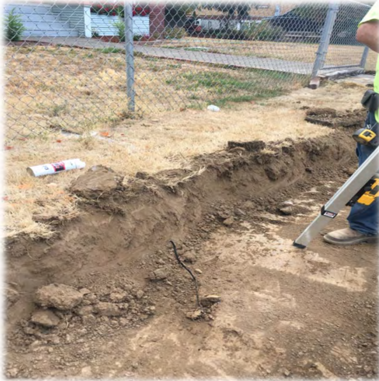
Excavation and grading
