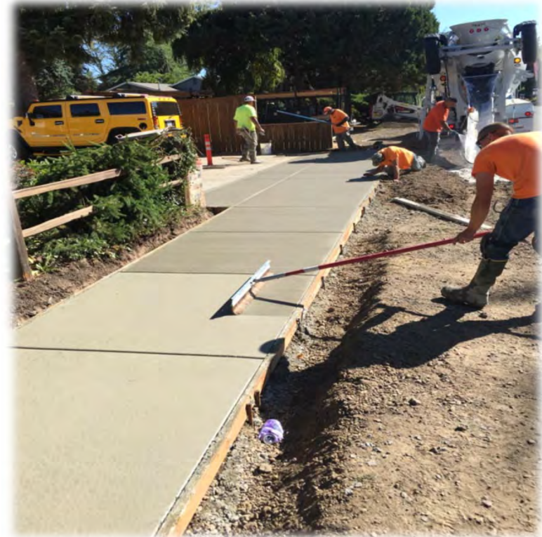
Concrete finishing
