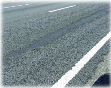
Raveling & Delamination
