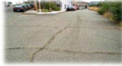
Cracking
