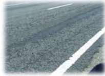
Raveling and Delamination
