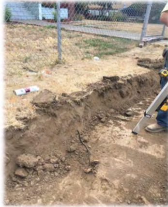
Excavation and grading
