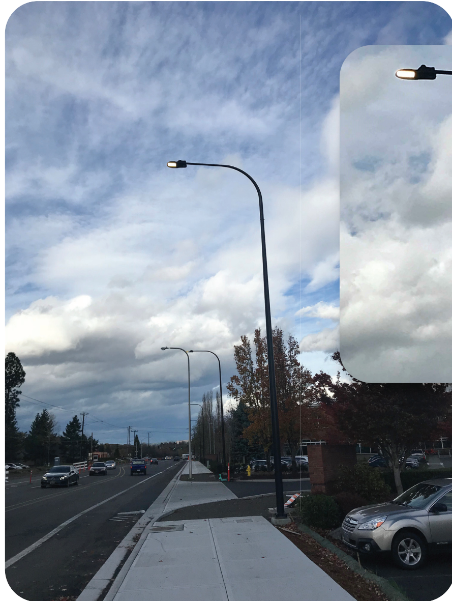
Street Light Example Shorter poles will be used on 198th
