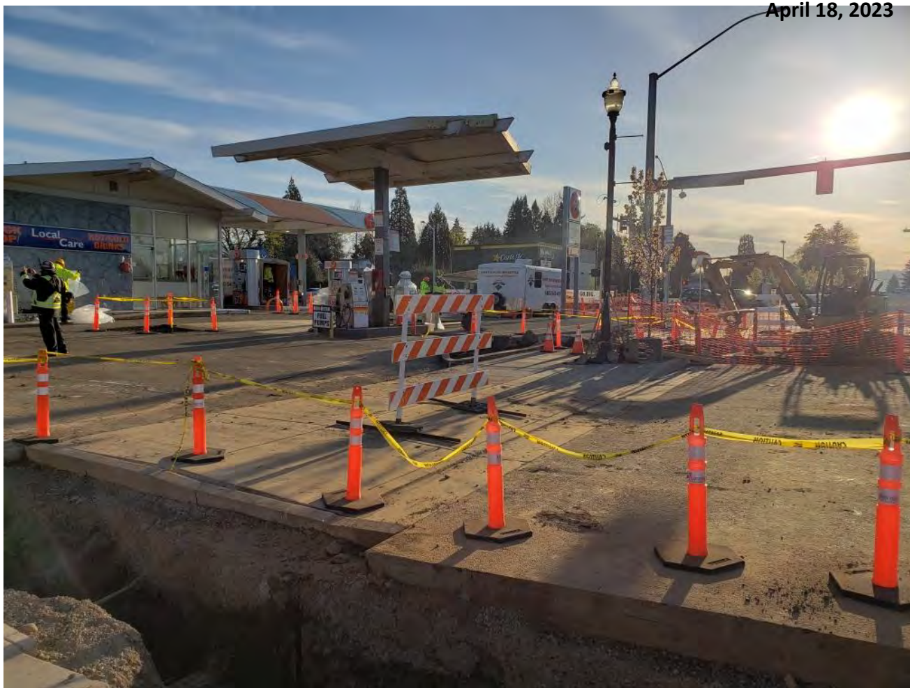
Cleanup on April 14, 2021, of a gasoline leak at the intersection of Main Street and Highway 99 in Monmouth. [Oregon Department of Environmental Quality]
