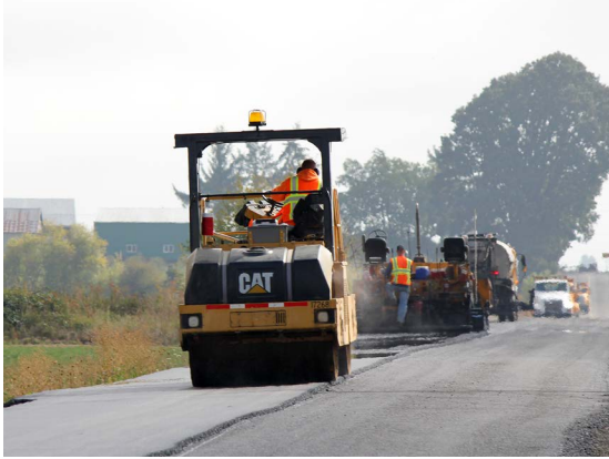
Washington County road maintenance crew
