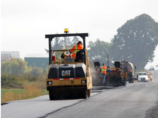
Washington County road maintenance crew
