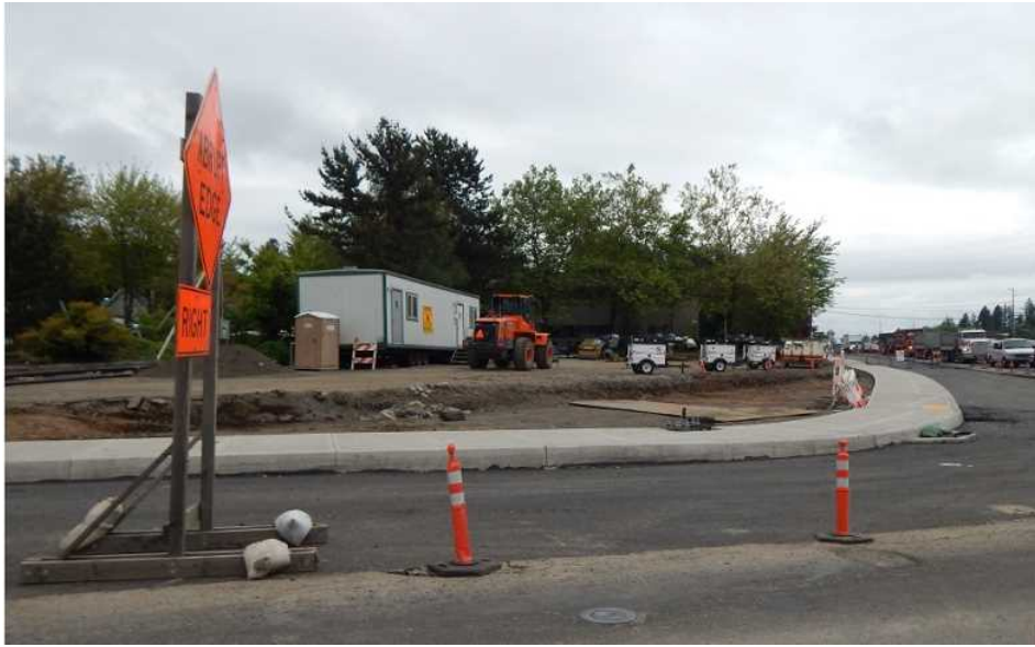
City of Tigard TDT funds leveraged state funds and county MSTIP funds to complete a capacity project at the intersection of Highway 99W, McDonald Street and Gaarde Street. The project added a second left turn lane onto Gaarde Street, a right turn lane onto McDonald Street, a southbound auxiliary lane on Highway 99W between Gaarde Street and Bull Mountain Road, and improvements to sidewalks, bike lanes and lighting in the vicinity. Image: Barbara Sherman, The Regal-Courier (Pamplin Media Group)
