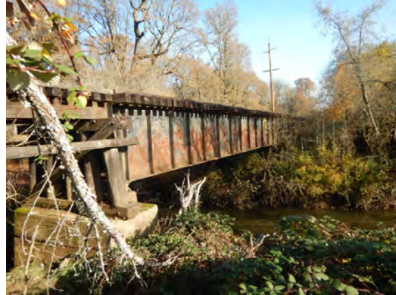
Steel Main Span
