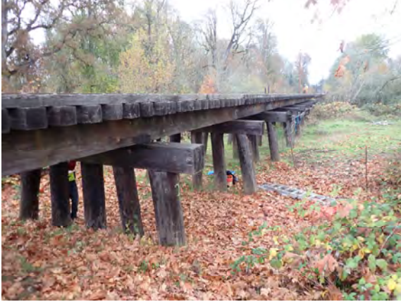
Timber Trestle Approach Spans
