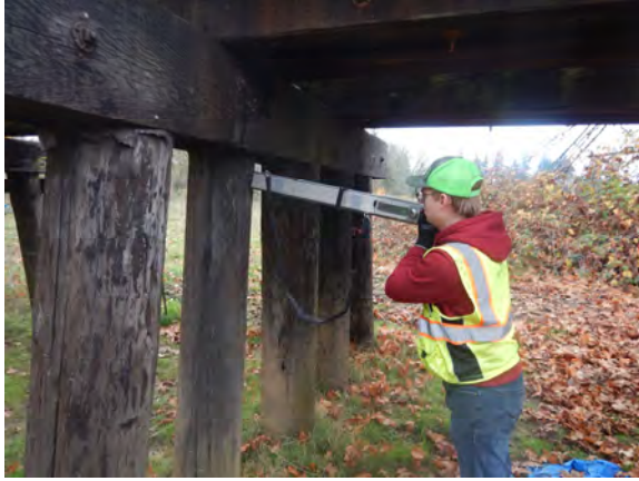
Resistance Drill Investigation of Timber
