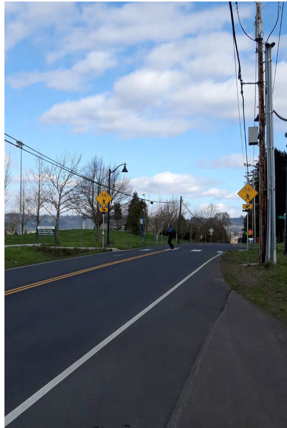
Mid-block pedestrian crossing at 173rd Avenue (Phase 4)
