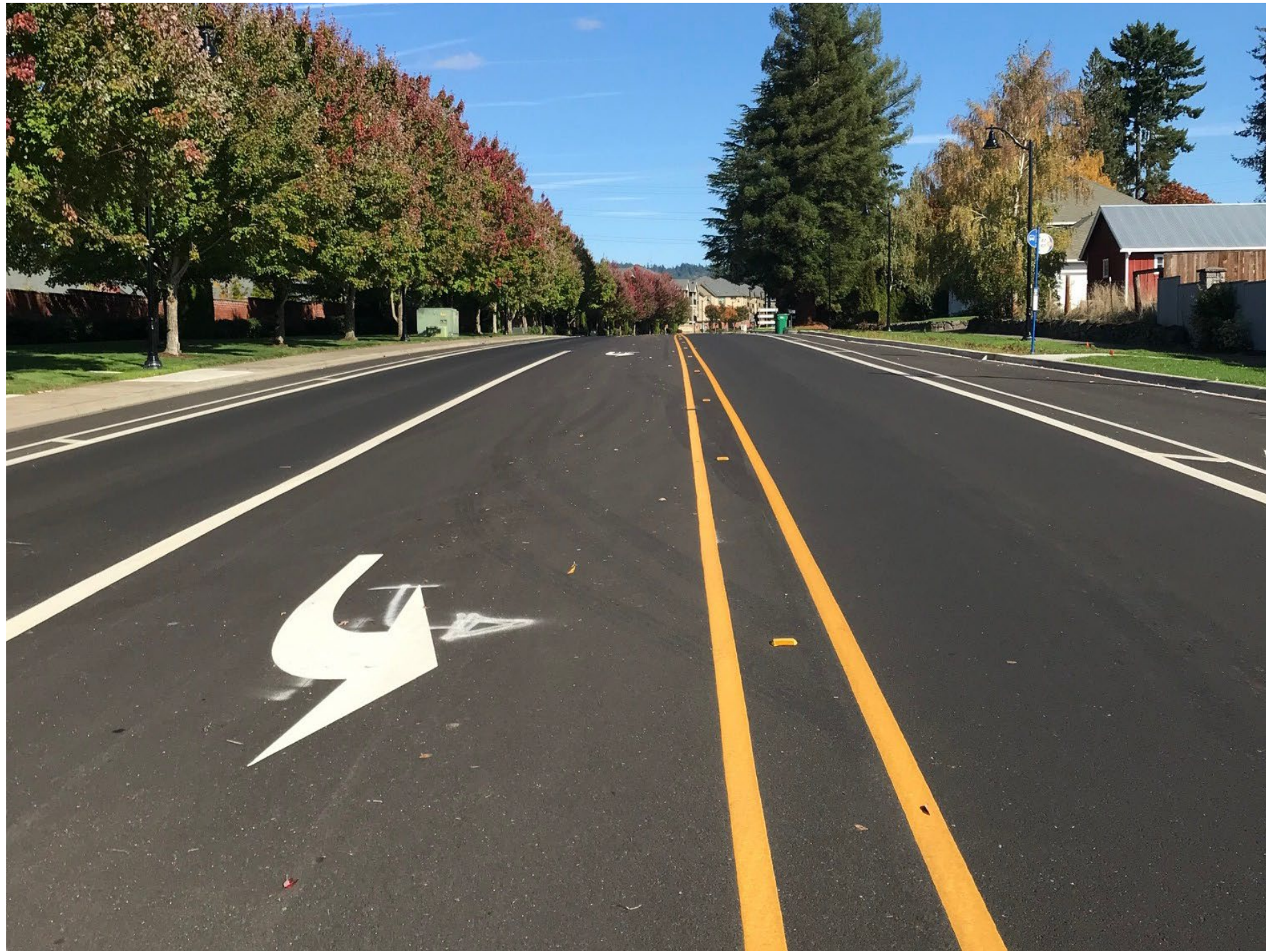
At Joss Avenue looking east
