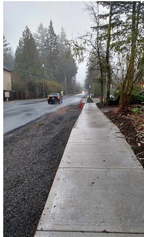
Taylor Street sidewalk constructed with Gain Share funding in December 2015.
