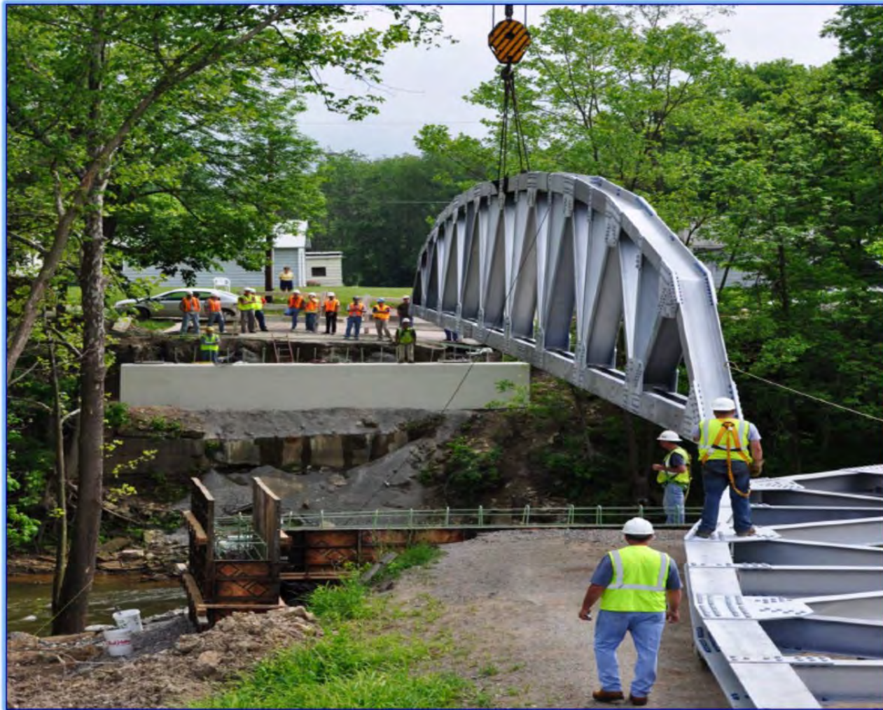
Bearing plates in position, truss is set in place
