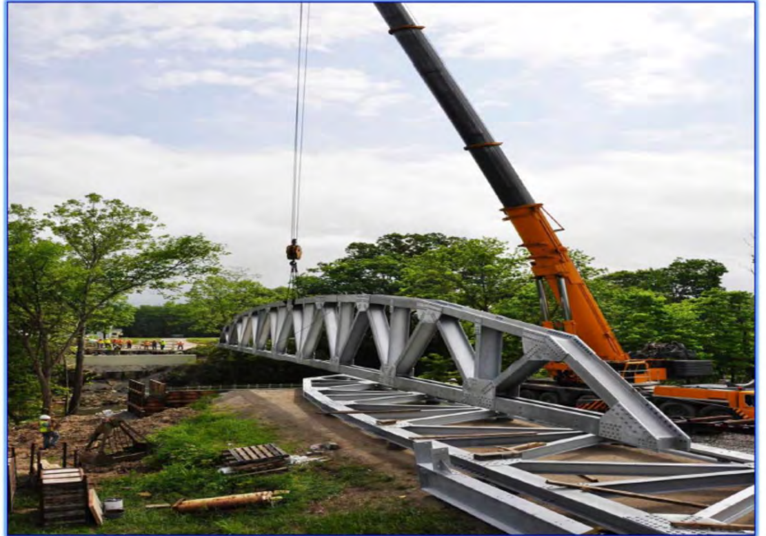
First truss is moved into position
