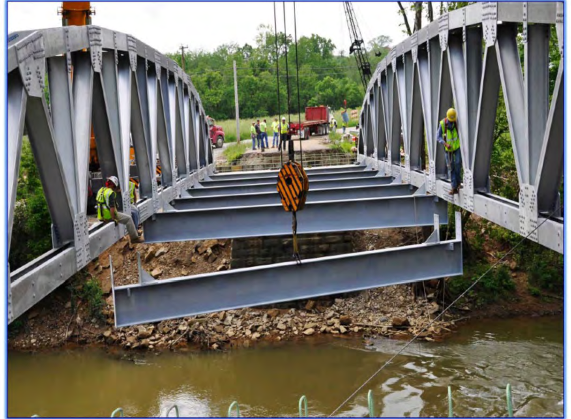
Once several floorbeams are installed, structure is stabilized
