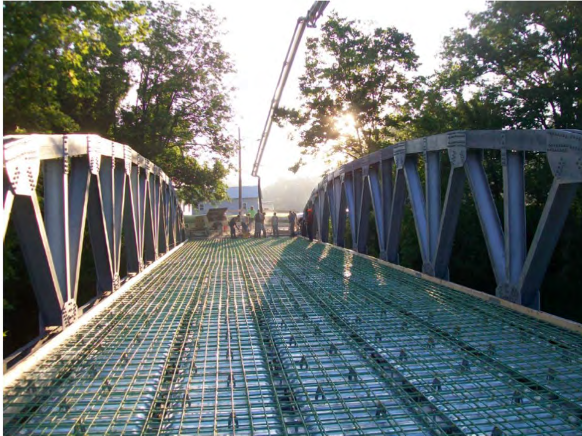
Reinforcement is placed and concrete deck is poured.
