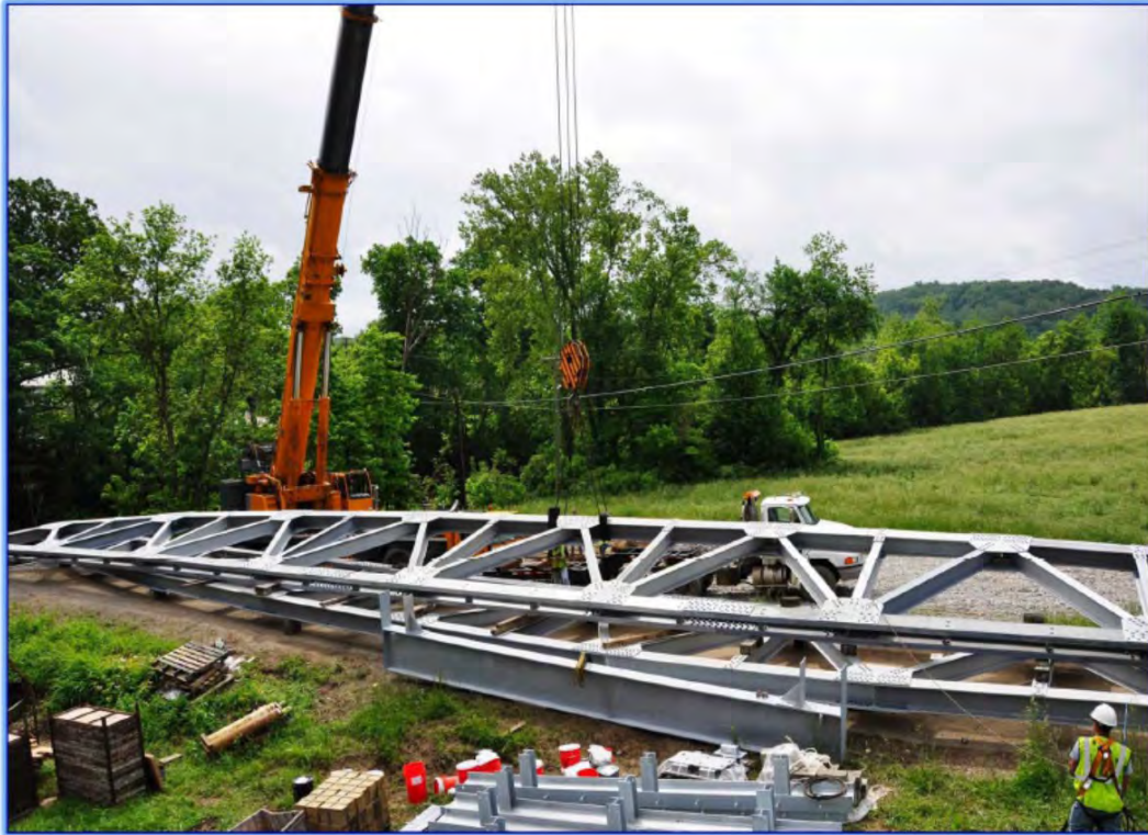
Truss sections are matched, assembled, bolts torqued
