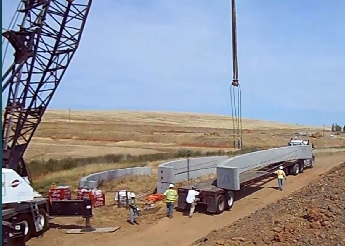
Arch Units are shipped to jobsite, picked and rotated to vertical
