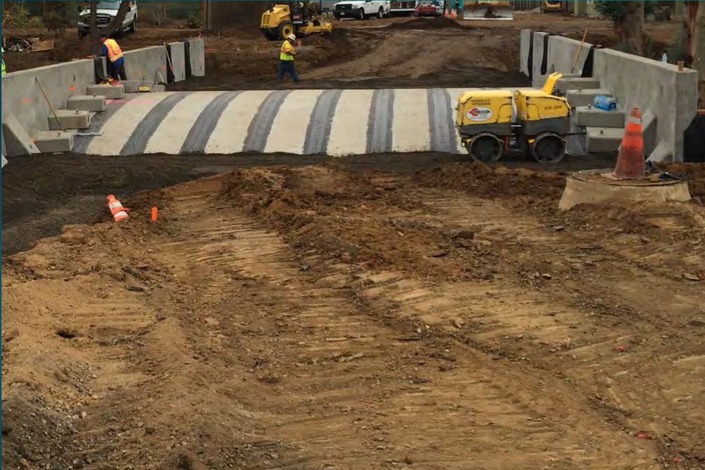
Structure is backfilled and end walls constructed
