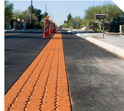
A cycle track in Tucson, AZ uses a textured buffer and bollards to provide a separated bikeway facility
