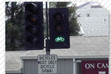
A bicycle signal with accompanying signage alerting bicyclists to obey the signal
