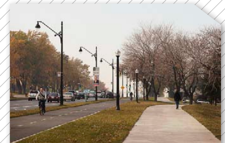
This two-way cycle track in Montreal, Quebec provides access to an adjacent park and is separated by a vegetated buffer
