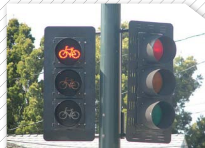
A bicycle signal in use in San Luis Obispo separates motor vehicle and bicycle movements
