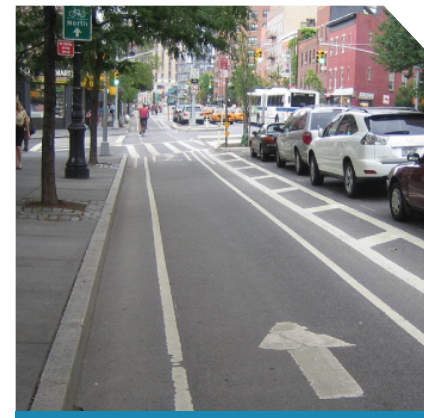
The 9th Street cycle track in NYC is on the left side of the street to avoid conflict with transit stops
