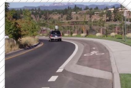
This raised and colored cycle track in Bend, Oregon vertically separates bicyclists and motorists
