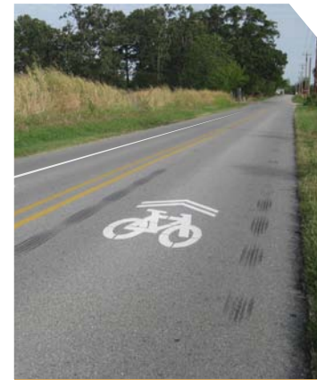
An uphill bike lane; downhill shared lane marking in a rural setting
