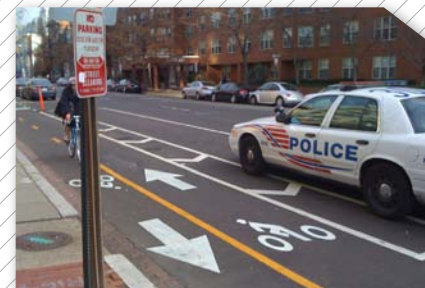
A new two-way cycle track facility in Washington DC is protected by a painted buffer and a parking lane
