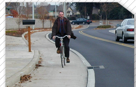
A raised cycle track in Corvallis, Oregon allows bicyclists to transition seamlessly into the travel lane when necessary
