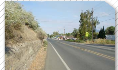
A paved shoulder on a rural arterial appeals most to recreational bicyclists traveling long distances
