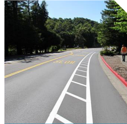
Buffered bike lanes increase the shy distance between passing motorists and bicyclists
