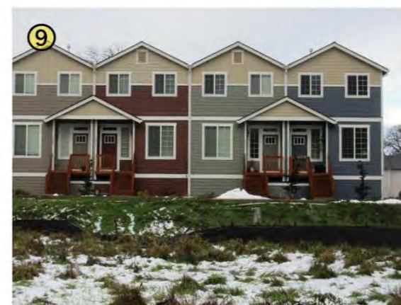
9 Many townhomes have raised entries and are tall compared to their older neighbors. Raised entries can pose challenges for seniors and people with disabilities.
