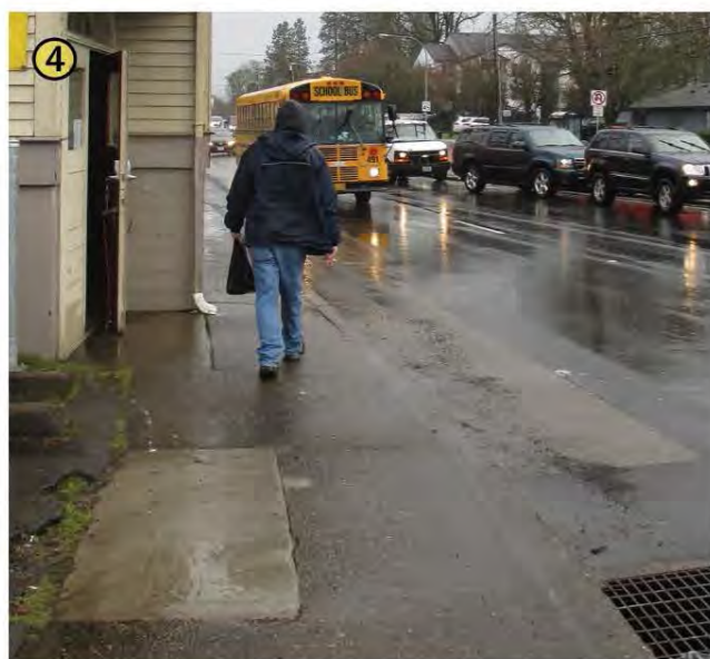
In commercial areas along TV Highway sidewalks are more common, although they are typically curb-tight. In places such as the west side of SW 185th Avenue, this makes for an unpleasant pedestrian experience—particularly next to the Grange, where the sidewalk narrows to 3' along a busy street with fast-moving traffic.
