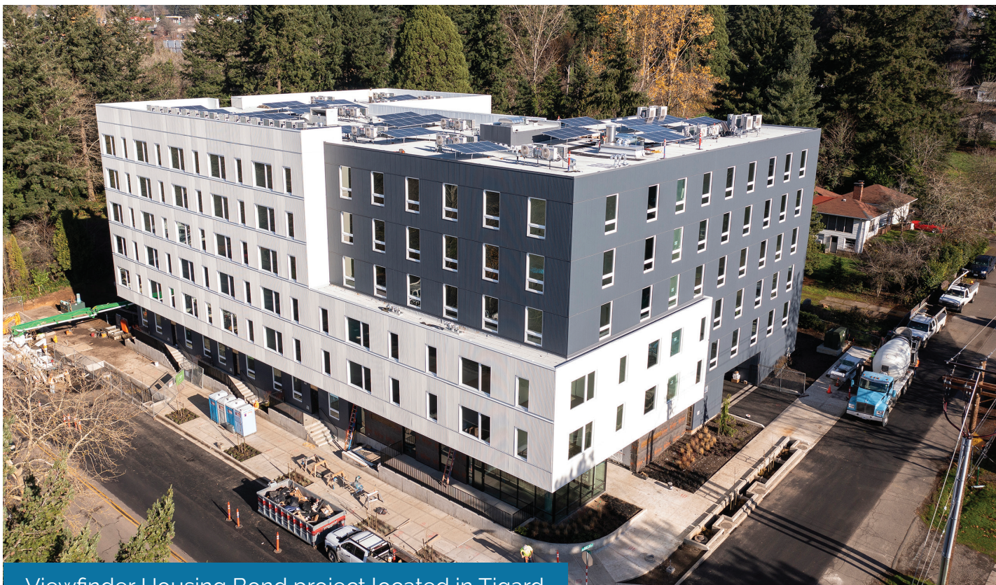
Viewfinder Housing Bond project located in Tigard
