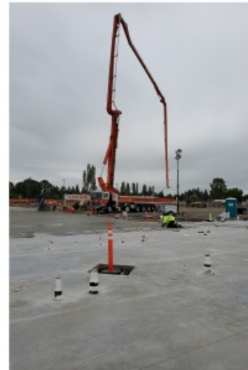
Taking advantage of a dry day to pour concrete-
