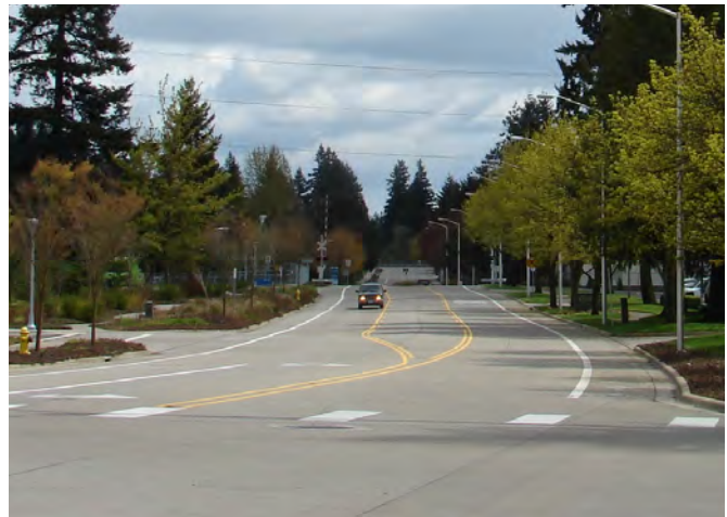
Example of a Collector - Barber Street looking east near SMART Central at Wilsonville Station transit center
