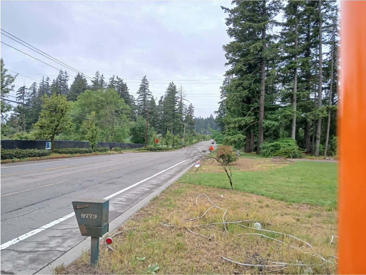
From site access looking west (single-use truck)
