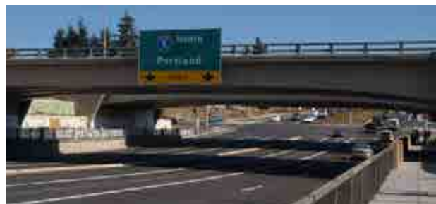
Looking east to the I-5/Wilsonville Road interchange.
